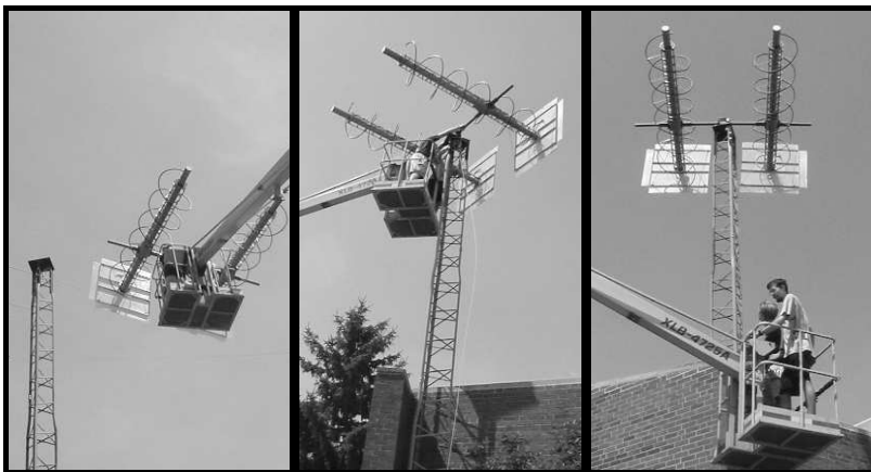
Lifting a pair of helical antennas.
